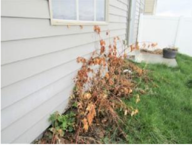
The shrubs along the back wall need to be trimmed to avoid contact with the structure and prevent damage to the property.
