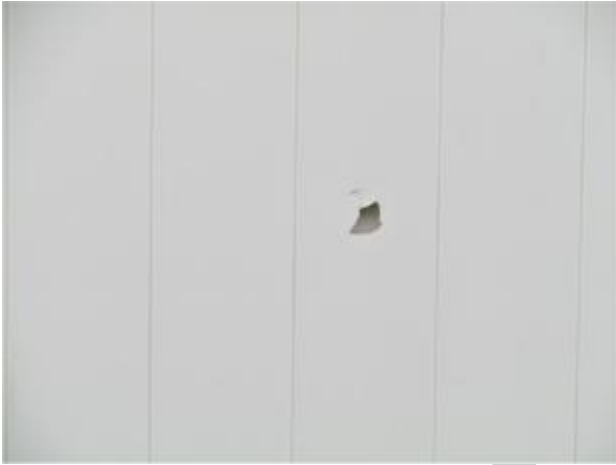
The fence around the backyard has damage.
